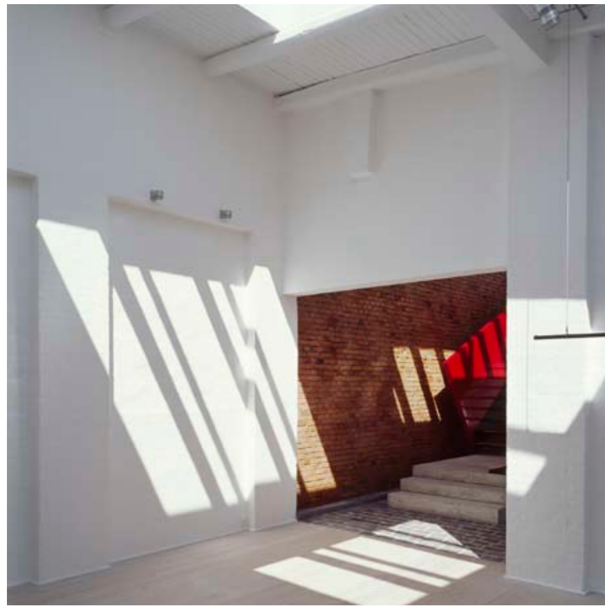
Left In the cloakroom and in the small hall, additional openings were created in the roof to allow daylight into the dark and gloomy workshop rooms.
