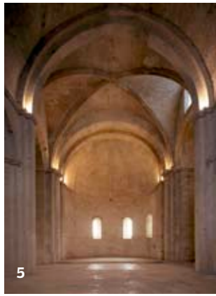
5. A compact, solid construction, like this at the Abbey of Montmajour near Arles, is typical of the Roman style of church architecture. Due to the kind of construction, there are only relatively small window openings through which light is barely able to penetrate. The church interior is usually only seen like this at twilight.
